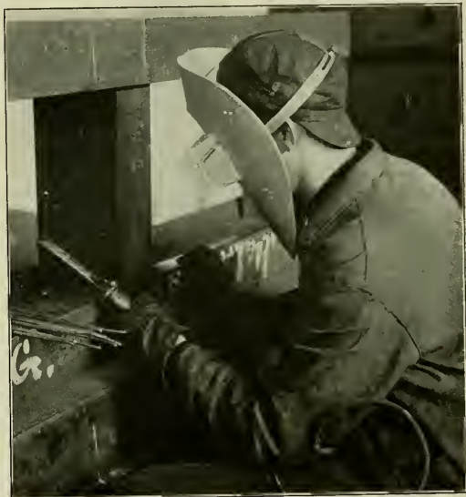
Operator Using Metallic Electrode.
